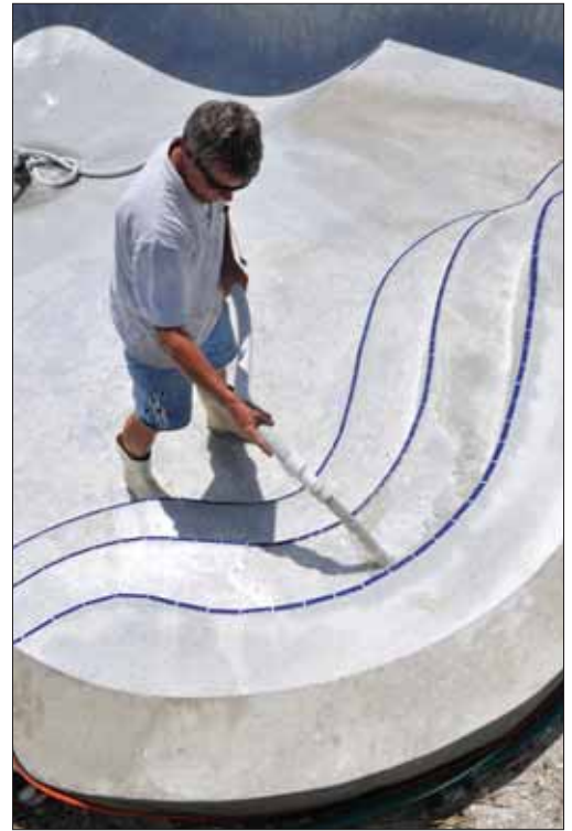
Above: Ralph doing acid wash. You can see the new cap. Below: Chaz helping with the form work
