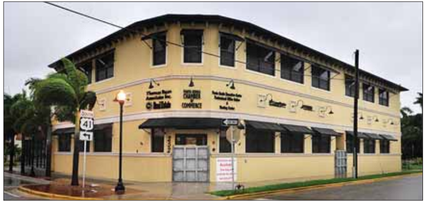
The Punta Gorda Chamber of Commerce's building installed these metal flood gates to hold back the high water anticipated in TS Fay but the waters never came. The new SunLoft Marketplace across Marion Ave will install similar protection. FEMA mandated flood protection for downtown Punta Gorda we'll likely see more of these contraptions installed around town.
